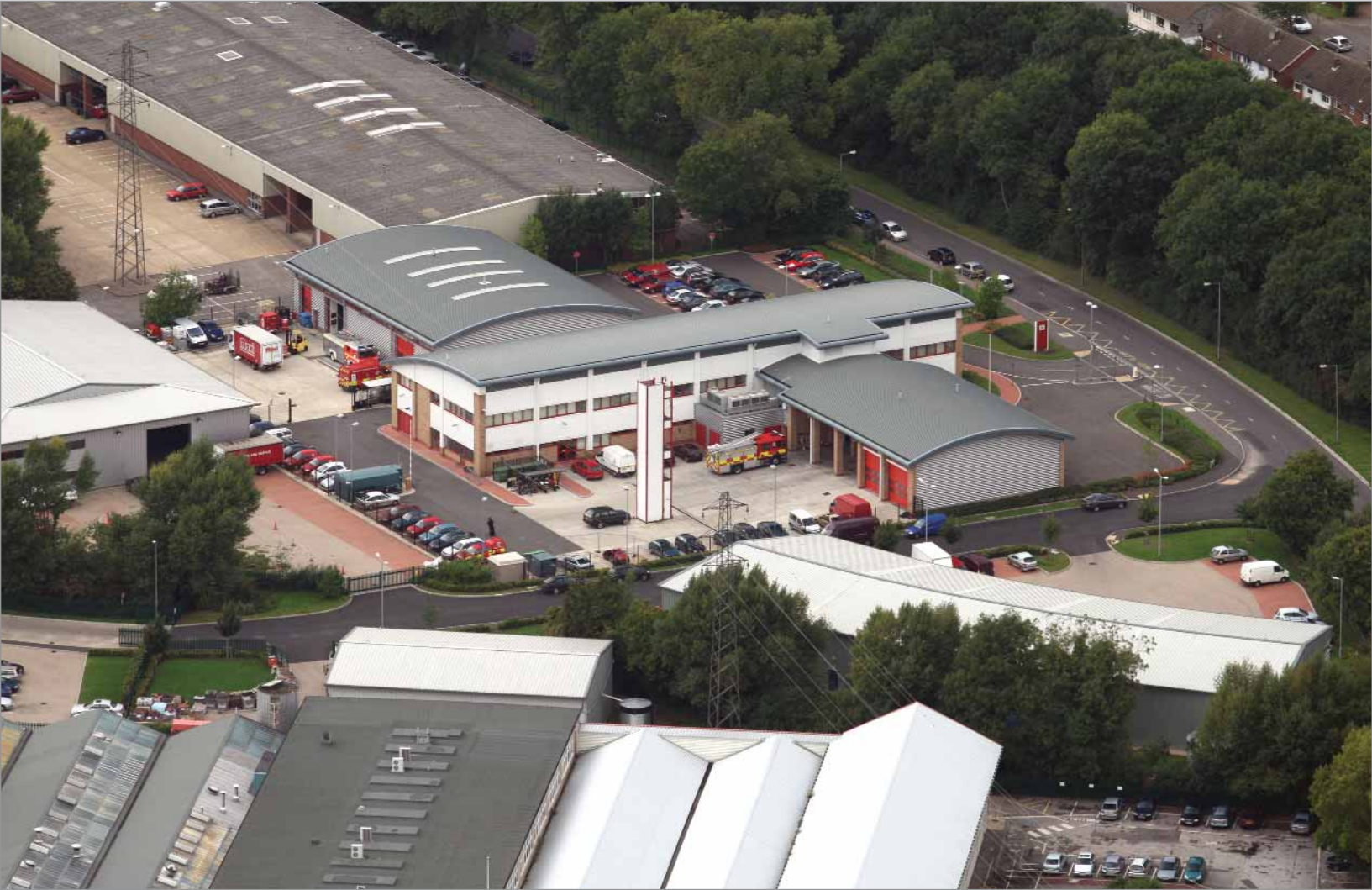
Brigade Headquarters and Aylesbury Fire Station seen from the air.
